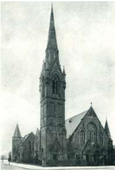
Fitzroy Avenue Church c1947
