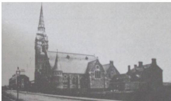
Fitzroy Avenue Church (c1877)
