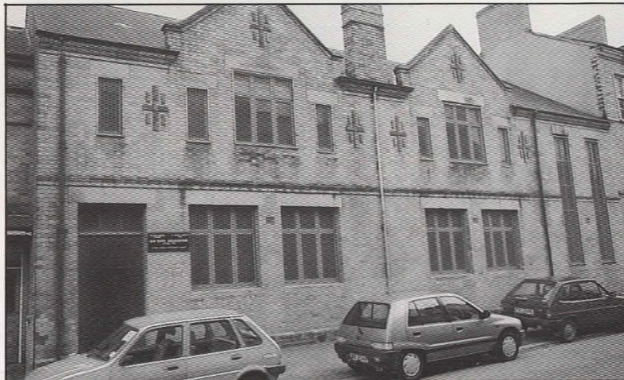
O.B. Hall - Fitzroy Avenue Opened 24th October 1908 "Where the work continues today".
